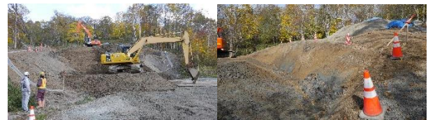
Photo.2 Construction yard foreground (left), excavation slope (right)
